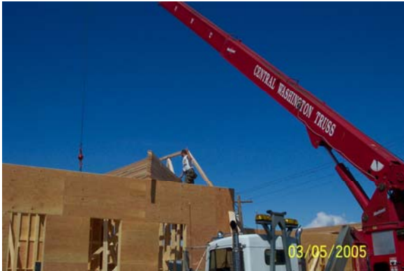
Rebuilding begins in 2005
